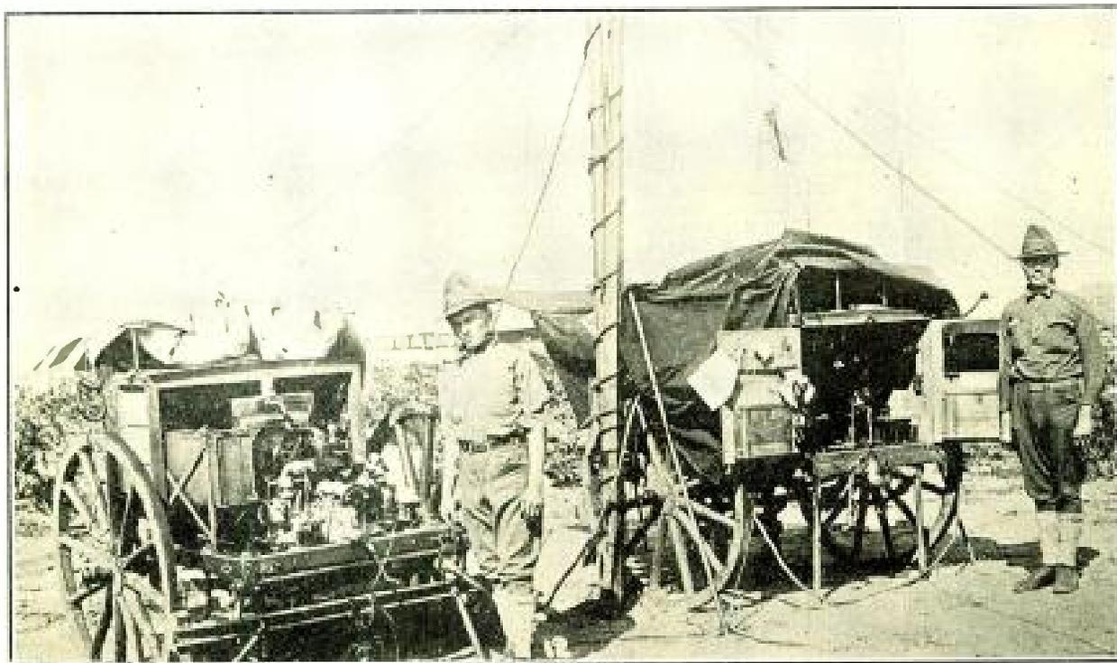
*A close view of the wireless equipments employed by United States troops when in the field. The apparatus is of light construction and can be erected and dismantled in a short time. It has great value as means of communication for the United States forces sent on the punitive expedition into Mexico against Villa because of the ease with which the wire telegraph lines can be cut*
