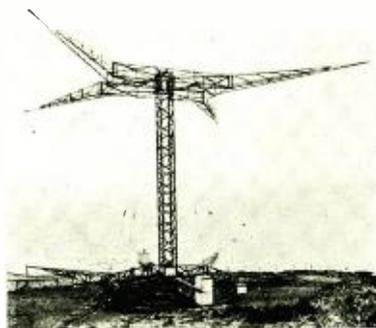
This is a "radio beacon" just erected at Inchkeith, an island in the Firth of Forth. It sends forth automatic directional compass bearings for the guidance of ships
