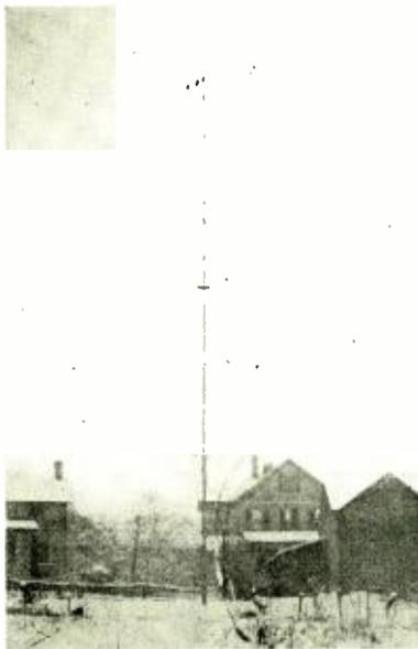
Antenna system of 2OM station consists of six wires on 20 ft. spreaders, 35 ft. x 80 ft. above ground, total length 75 ft. natural period
