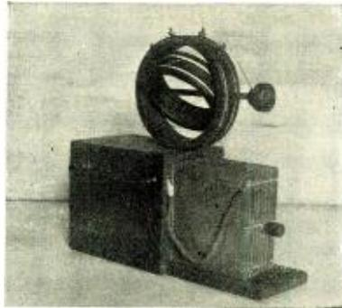
Figure 3. Home-made variometer and variable condenser
