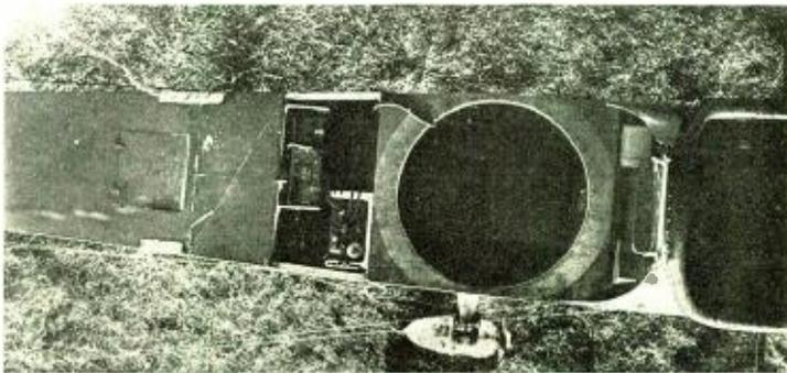
Looking down into the radio cockpit. The wind-driven generator is shown on the starboard side. Transmitting and receiving equipment is seen in the space aft the cockpit. Boxes of spare tubes are carried in the forward compartment
