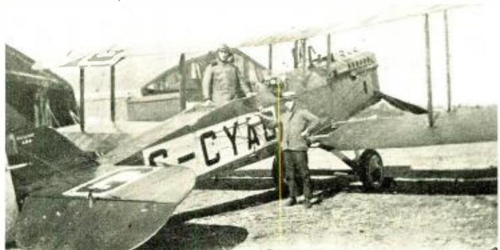
Radio observer in DH-4 airplane, about to start on his daily forest patrol. The man on the ground has his hand on the 600-volt generator that supplies current to the radio transmitter
