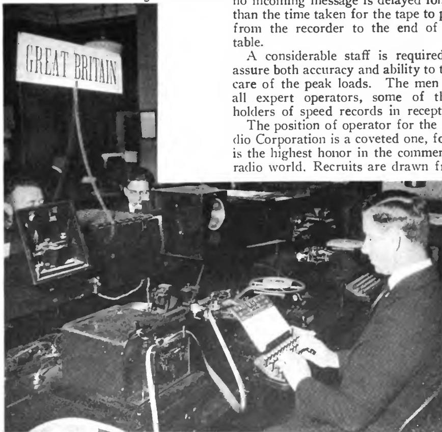
Close-up of transmitting side of English circuit, showing operator at Kleinschmidt perforator. The tape from this passes through the Wheatstone transmitter at the left. One perforator is capable of from 75 to 80 words a minute, and in case greater speed is required, a second operator uses the spare perforator seen at the right
