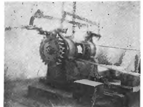
Figure 4. Belt-driven rotary spark gap of the Colomb Béchar spark transmitter
