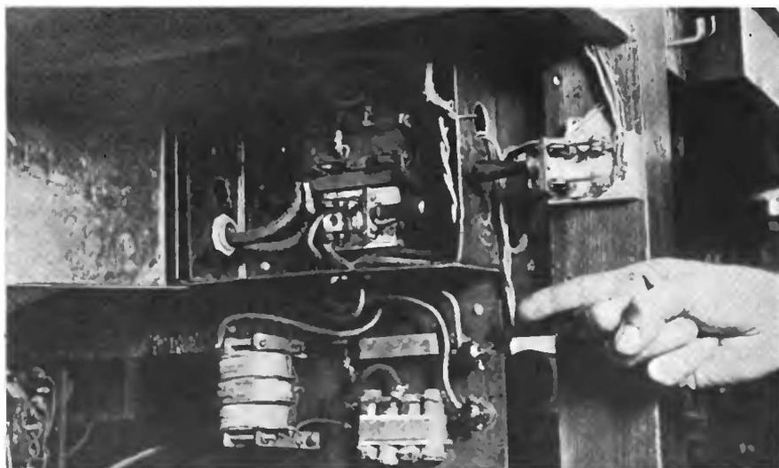
This little device, tucked away under a table in the operating room at WJZ, played its part in the successful transmission of the baseball results. It consists of resistance coils and transformers and its duty was to eliminate distortion on the wire line from the Polo Grounds to the broadcasting studio.
