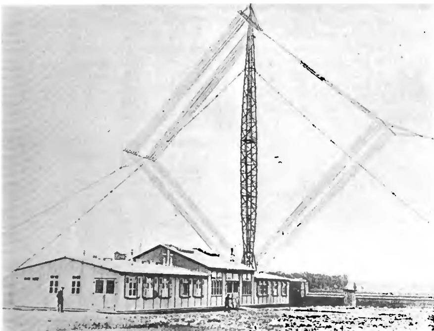
This is not a direction finder, as might be expected, but a novel form of transmitting antenna at the new German wireless station at Oranienburgerstrasse. Signals from this antenna are so strong as to be audible not only in all parts of Europe but in North America and in Asia
