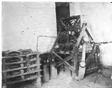
Figure 2. The antenna oscillatory transformers at the Colomb Béchar wireless station
