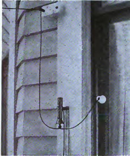
Figure 3—Effective lightning arrester installation
