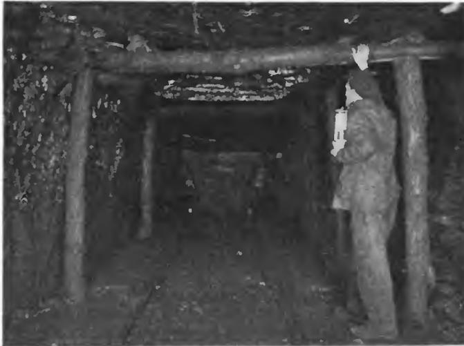
Cross-bar rigging to insure safety to miners engaged in working loose strata—the dangers of which may be further guarded against by use of radio
