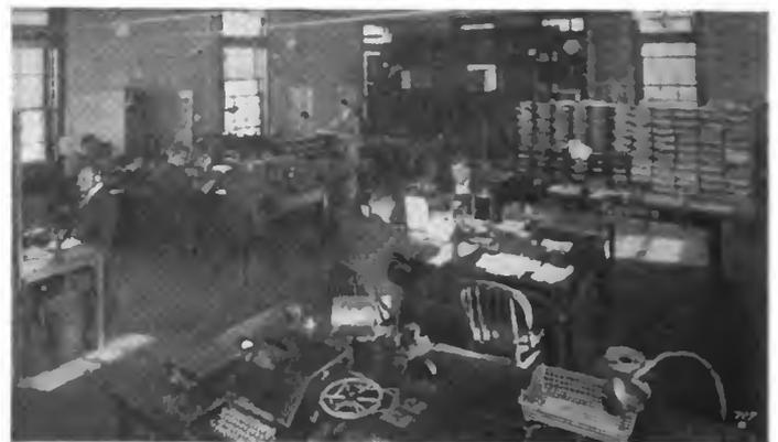
Another view of the operating room. The machine in the immediate foreground, with keys, is a perforator for the tape used in high speed transmission, and is similar to the device used on the "*Majestic*"
