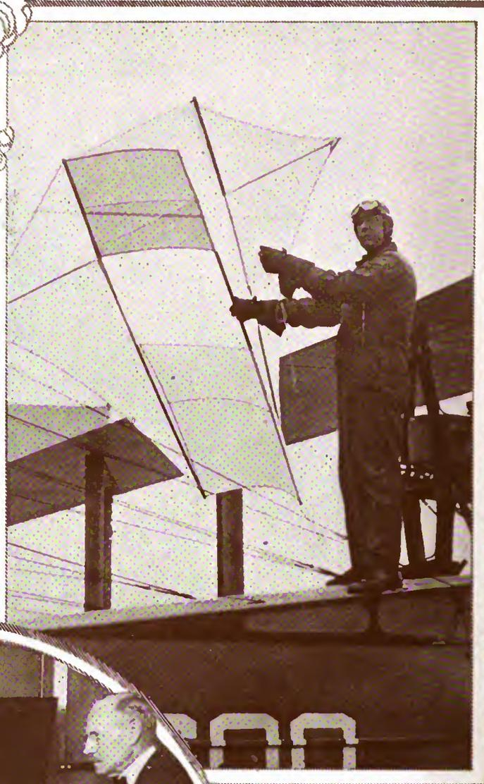
*While somewhere out at sea a naval aviator flew this kite, in order to hoist a radio antenna from his floating seaplane*
