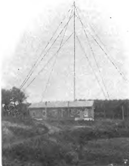
The operating building at Chatham, with one of the local aerials used for work on 600 meters. The telegraph poles faintly seen back of the structure support one end of a receiving antenna a mile long
