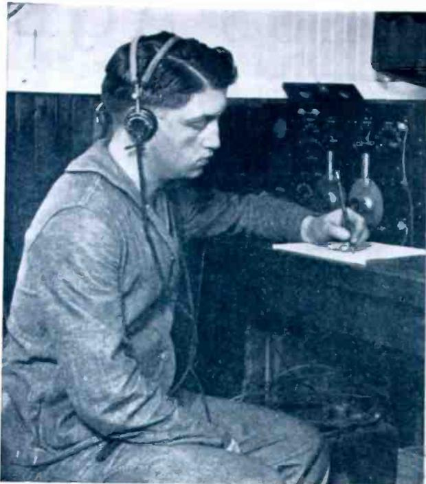
Naval operator at the radio station at Lakehurst. The receiving set shown is the navy type employed at most of the naval land stations
