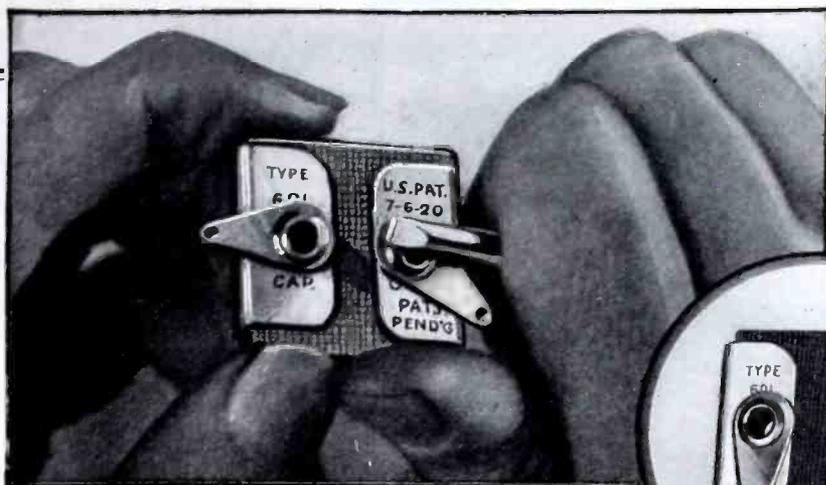
If Dubilier Micadons are to be connected by means of the eyelets and screws, swing the extension soldering tabs aside or clip them off.
