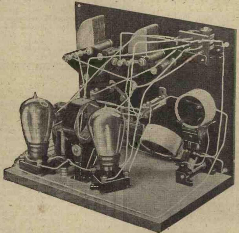
*In laying out a set, "make sure there is adequate clearance between the valve and other parts of the set to allow of vibration."*
