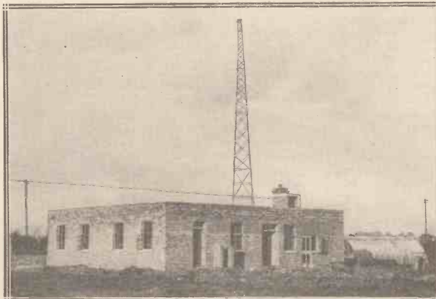
Radio constitutes both the eyes and the ears of the Air Force, and this new station under construction at Mitcham for the Air Ministry will play a great part in the future development of aviation.
