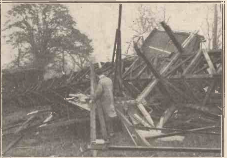
All that remained of the 210-ft. mast and the wireless equipment of the Radio Research Board station at Ditton Park after a devastating fire which broke out in the laboratory. The mast, blazing furiously, crashed down on the main shed, forming a terrible and majestic spectacle.
