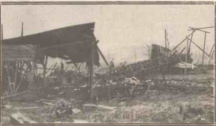
The result of a disastrous fire that broke out at the Ditton Park laboratories of the Radio Research Board. The station was completely gutted and the 210-ft. mast crashed in a sheet of flame.
