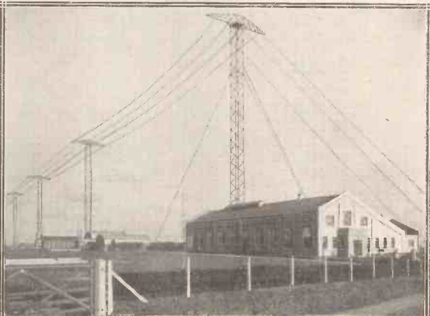
Britain leads the way in short-wave transmitting services, high-speed communication being possible between this country and all the main points of our far-flung Empire. This photo shows the Beam transmitter aerial system at Dorchester, whence messages are sent to Rio de Janeiro and New York.
