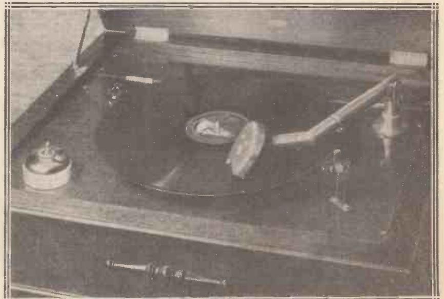
The turntable, on-off switch, and B.T.H. pick-up which form the top section of the electric gramophone.
