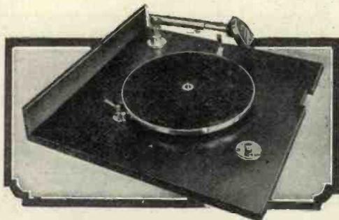
How the turn-table is arranged in the Gramophone Three. The pick-up and tone-arm used in the original set were of B.T.H. manufacture. Other suitable alternatives can, of course, be used, but care must be taken to get the proper tracking
