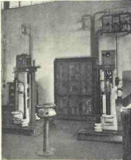
Switchgear at the new Leipzig broadcasting station. The output stage is duplicated in case of breakdowns
