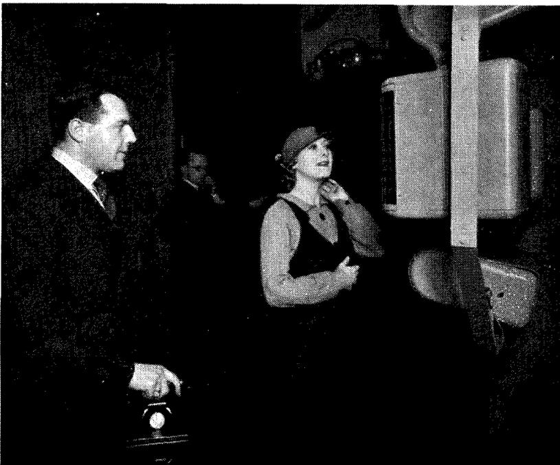
High-definition scanning by the moving-spot process in a modern television studio. Alma Taylor is seen here being "shot" in close-up at the Baird station
