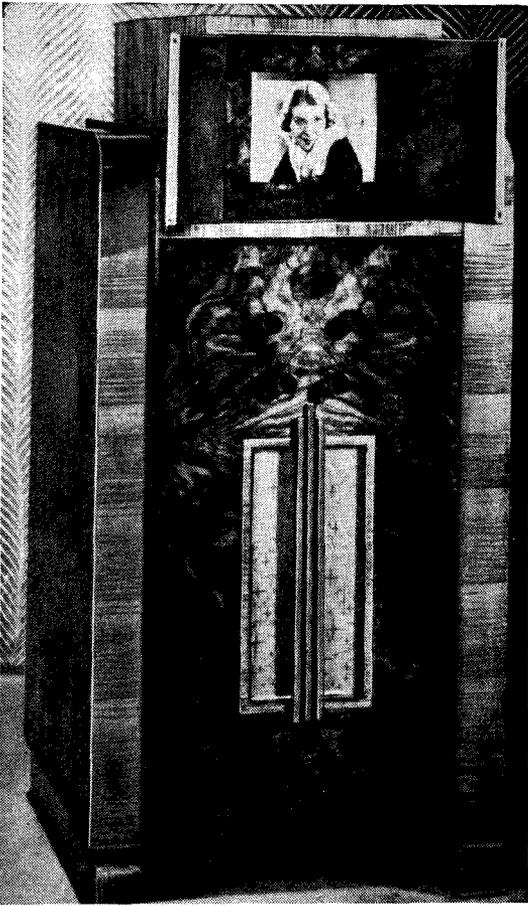
Also on show in Berlin: a Philips television set. This, too, is of the twin-channel type and employs a cathode-ray tube for viewing
