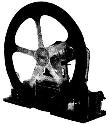
*A simple form of disc receiver operating on the spiral-perforation system described by Mr. Harris in this article*
