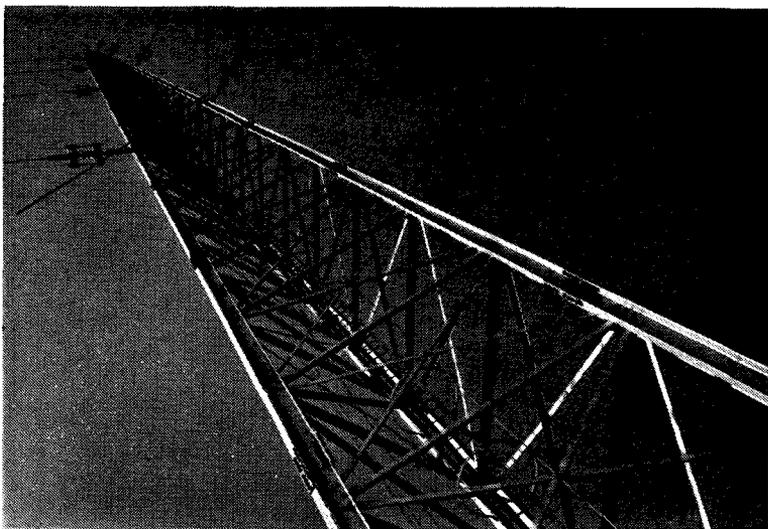
An impressive photograph of one of the new aerial masts at the Hilversum station. The mast is of the latest type and is actually the aerial—no wires being employed at all
