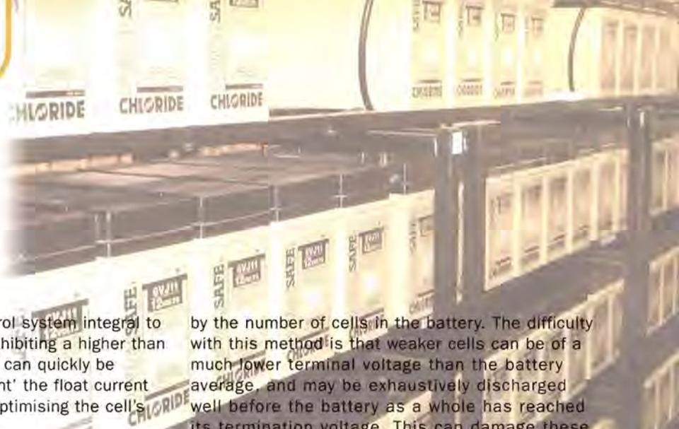
With the SoC intelligent control system integral to the cell however, those cells exhibiting a higher than specified float terminal voltage can quickly be detected and a system to 'shunt' the float current around the cell devised, thus optimising the cell's terminal voltage.
