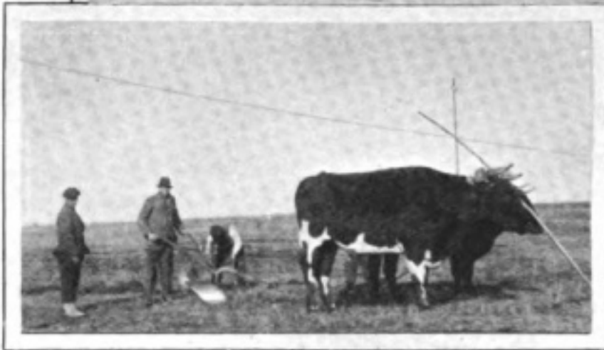
PLOUGHING IN EARTH WIRES.
