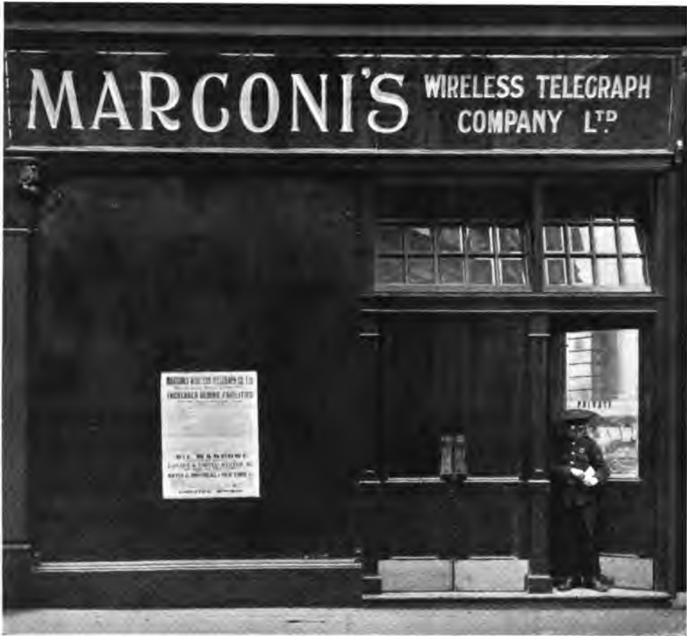
Exterior of Fenchurch Street Office.
