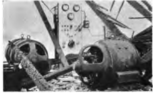
The Wrecked Generators at Duala.
