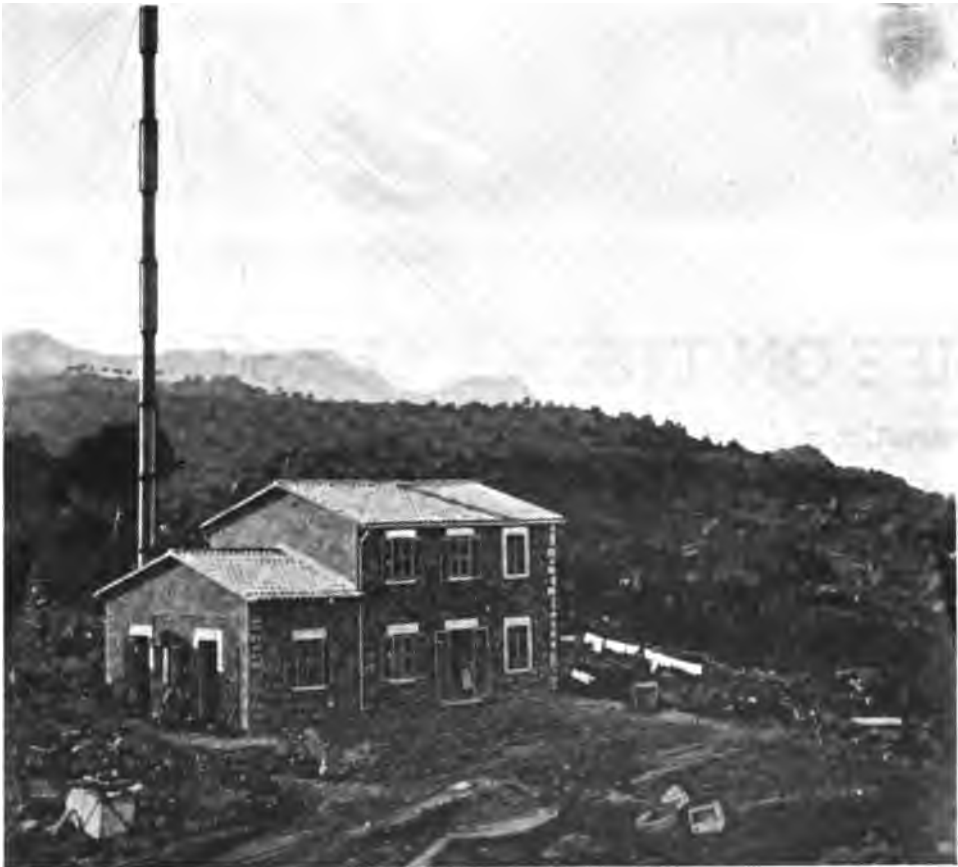
Wireless Station at Sóller, showing base of Sectional Steel Mast.
