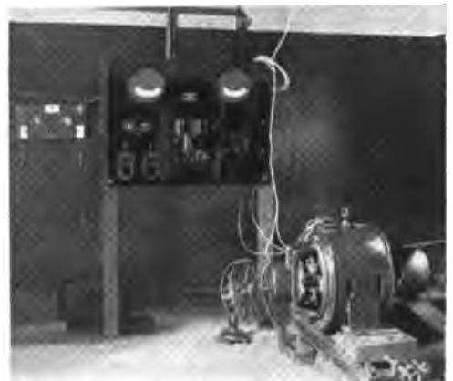
The Dynamo and Switchboard for charging Accumulators.
