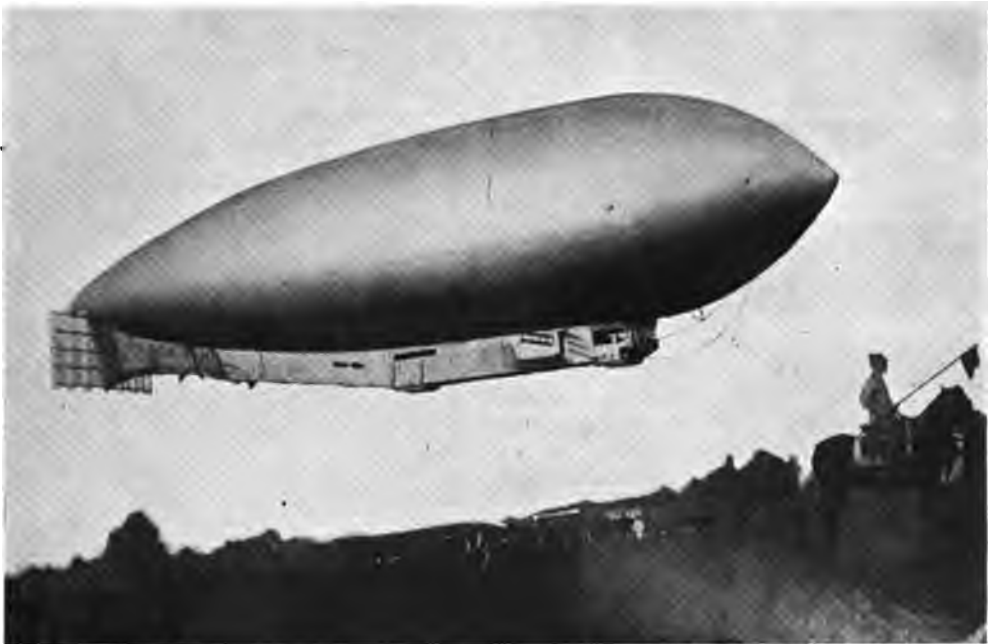
The "Forlanini" type of Airship used by our new Italian Allies. The car is a rigid structure forming part of the actual balloon.
