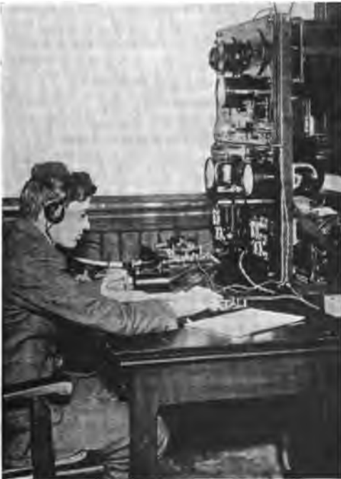
Wireless Installation at New York Fire Station.
