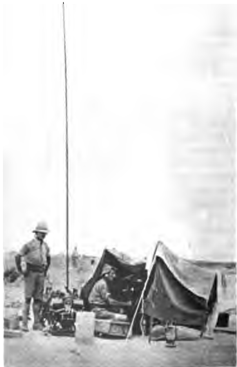
Pack Wireless Station.
