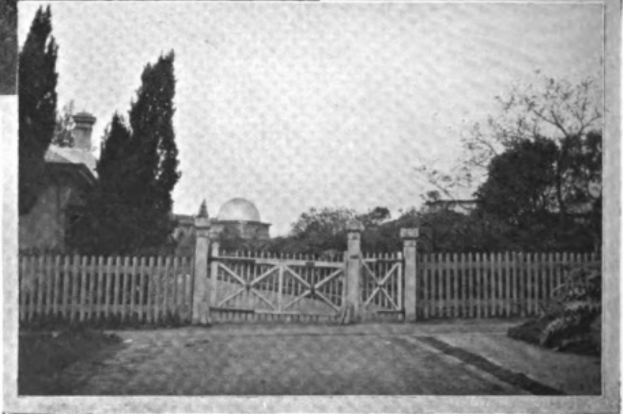
THE MELBOURNE OBSERVATORY, CONNECTED BY WIRE WITH THE WIRELESS STATION NEAR BY.
