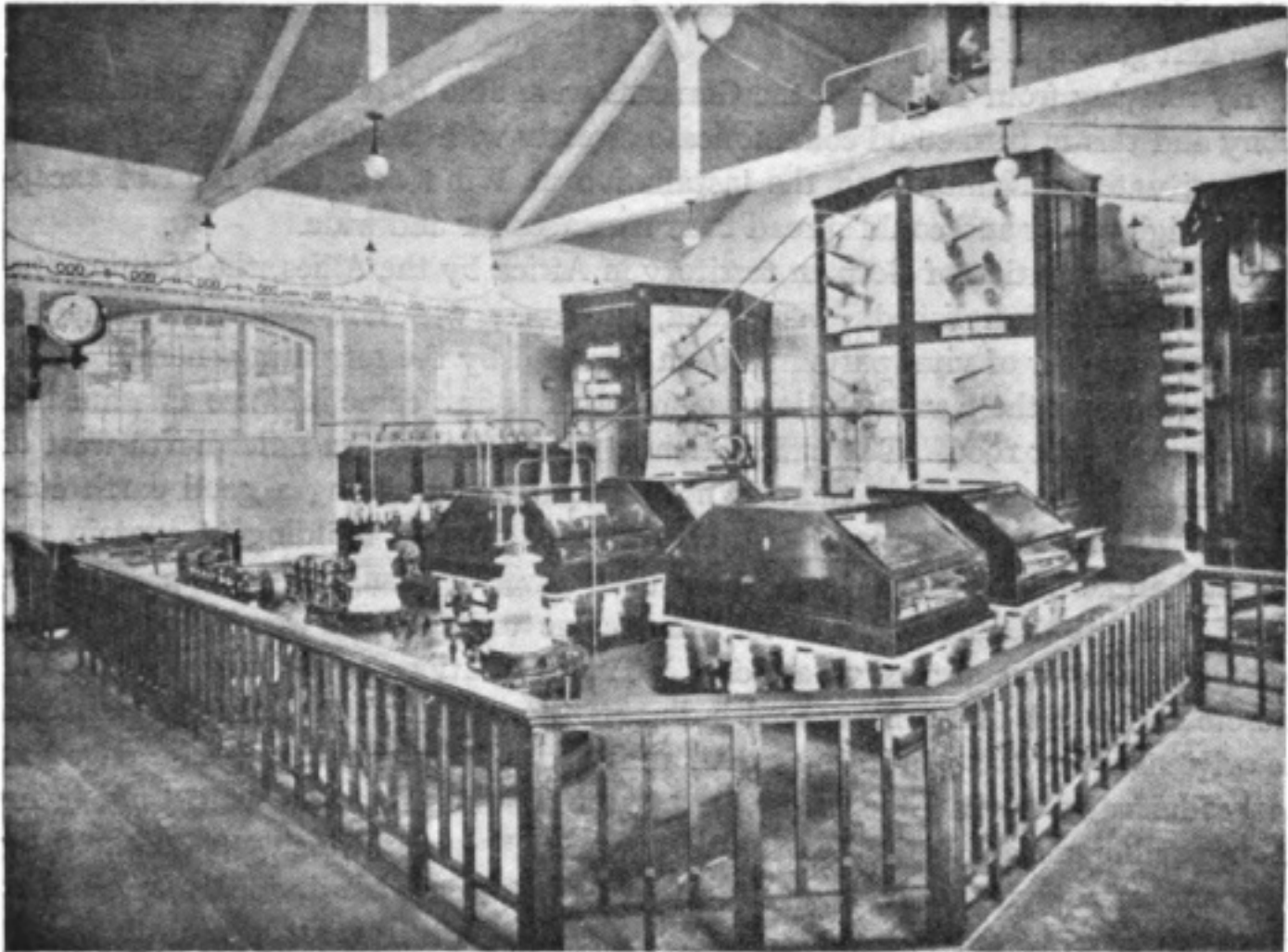
THE TRANSMITTING APPARATUS AT NAUEN.
