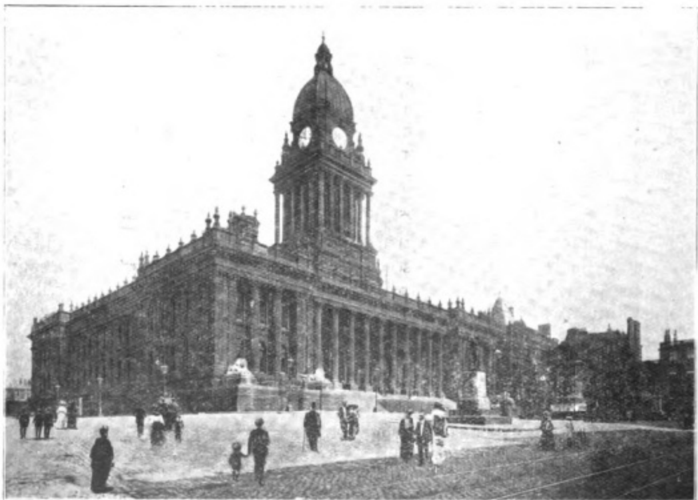
▲ The Town Hall, Leeds. Special facilities are being offered to wireless students in this city ; for particulars of the scheme see pages 567-8.
