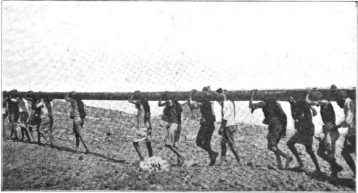
CARRYING A MAST SECTION TO THE STATION SITE.
