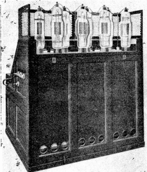
Fig. 5. Rear view of transmitting unit.
