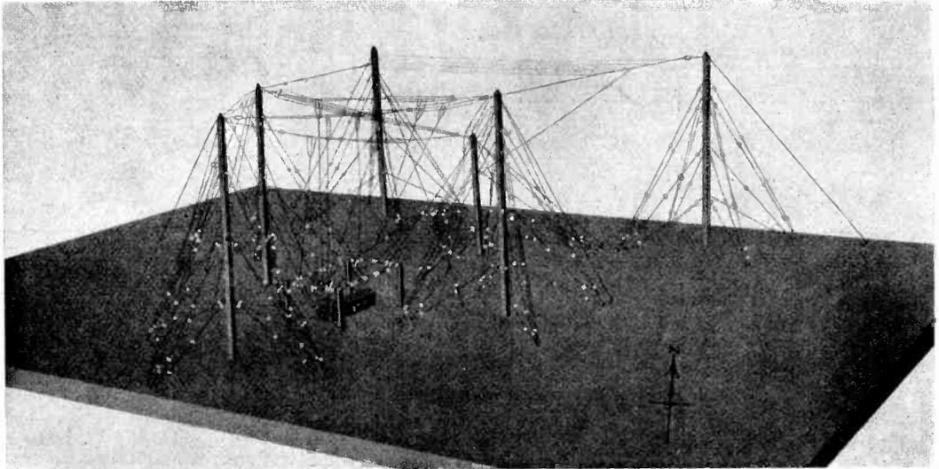
*Fig. 2. Model of the Aerial System showing the arrangement of a number of separate aerials.*
