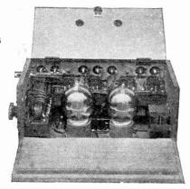
The Loud Speaking Equipment is used in conjunction with any good type of Valve Detector Set for amplifying radio telephone speechor music.
