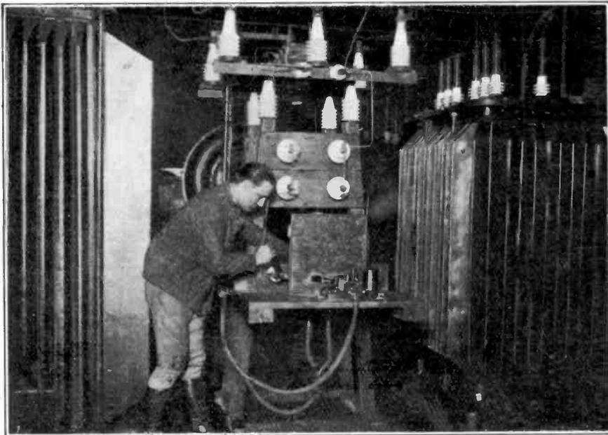
*Fig. 4. The pneumatic relay, used for signalling in the high tension circuit. The arc caused by breaking the circuit is extinguished by compressed air.*
