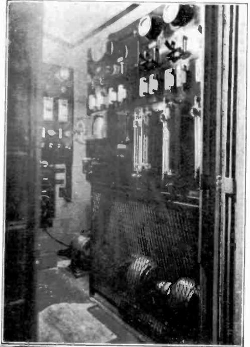
*Above. — The motor generator and main switch-board at the charging station of The Park Motor Co., Ltd., in Wells Street, S.W.*
