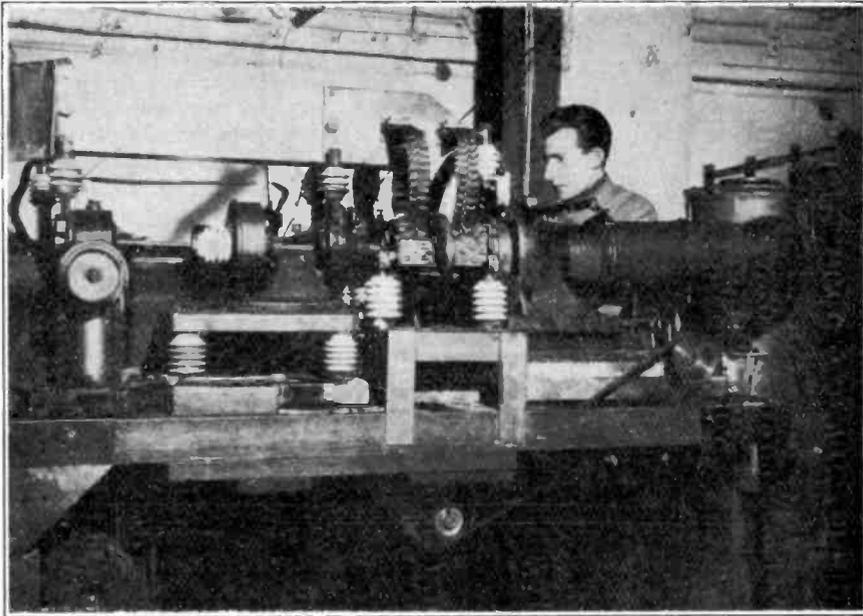
*Fig. 3. The spark gap, with ventilated revolving electrodes, and arranged so that the total sparking distance is synchronously broken down by the discharge a condenser bank separate from the main oscillator.*
