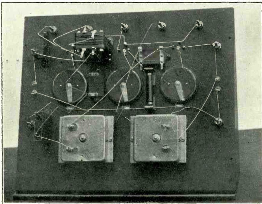
*The underside of the panel, showing the arrangement of the components and the wiring.*
