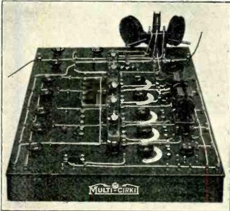
The arrangement of the components permits of particularly short wiring. It is a valuable instrument for trying out and investigating the many new circuits which have recently been developed. The makers are the Clarophone Radio Co., Palace Chambers, Bridge Street, Westminster, S.W.1.
