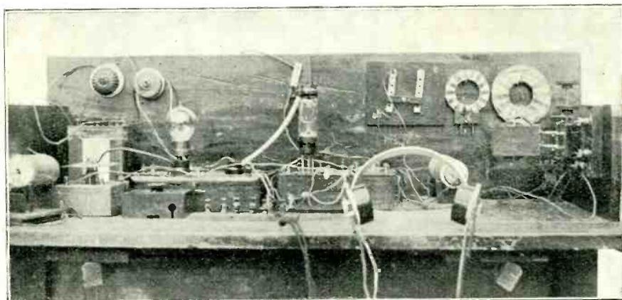
One of the successful attempts in the Transatlantic Tests was that of Mr. F. Walker, of Feltham, Middlesex. Our illustration shows the set used, which comprises a detector valve with high frequency amplifier. The home-made coil holder appears on the extreme right and the H.F. transformer and condenser on the left. The tuning condenser will be seen behind the telephones, to the right of the detector panel.
