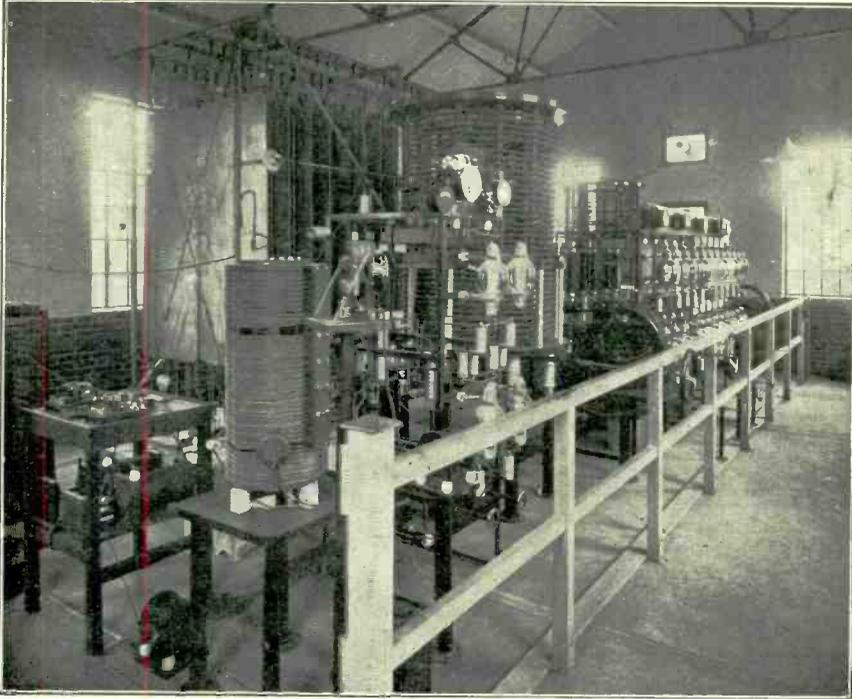
*The valve transmitter at the Ongar Station. It is interesting to note the handles for remote control and the compact layout of the apparatus.*
