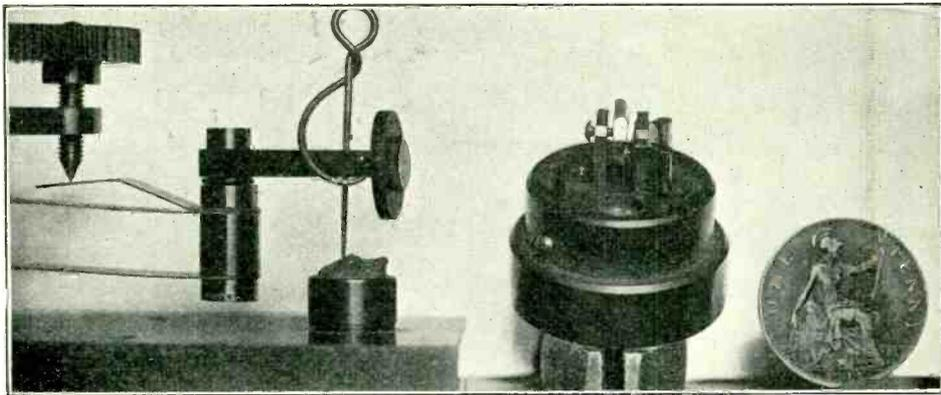
Fig. 1. The relative dimensions of the two types of crystal detectors are shown in comparison with the size of a penny.
