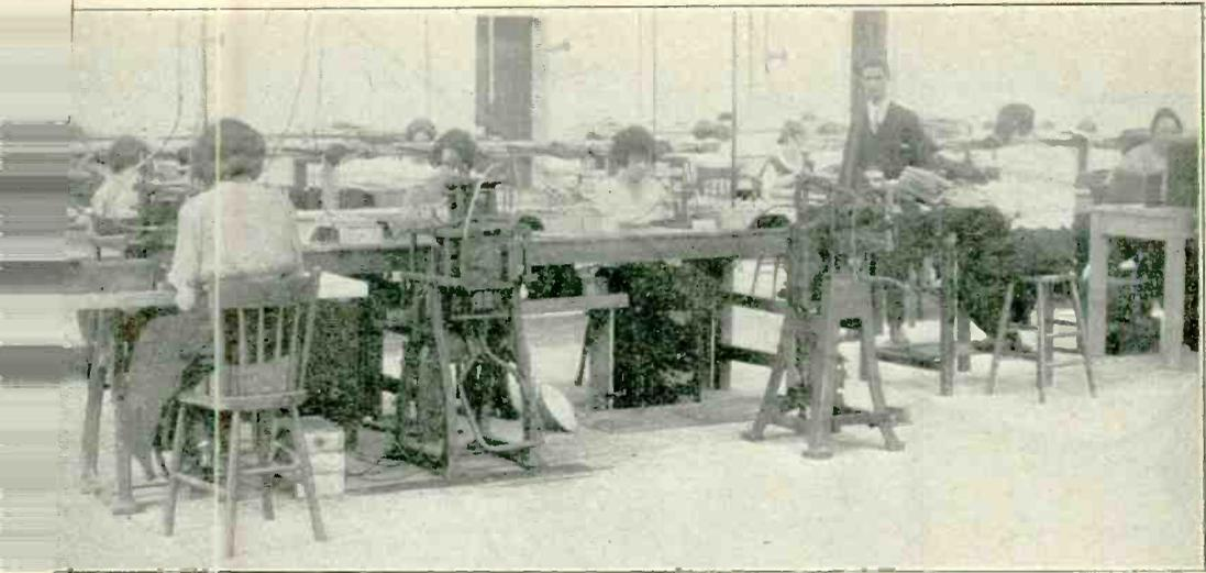
*One corner of the valve assembly room. Here the filament is connected to its supports, the grid is wound and mounted and the anode is welded to its support.*
