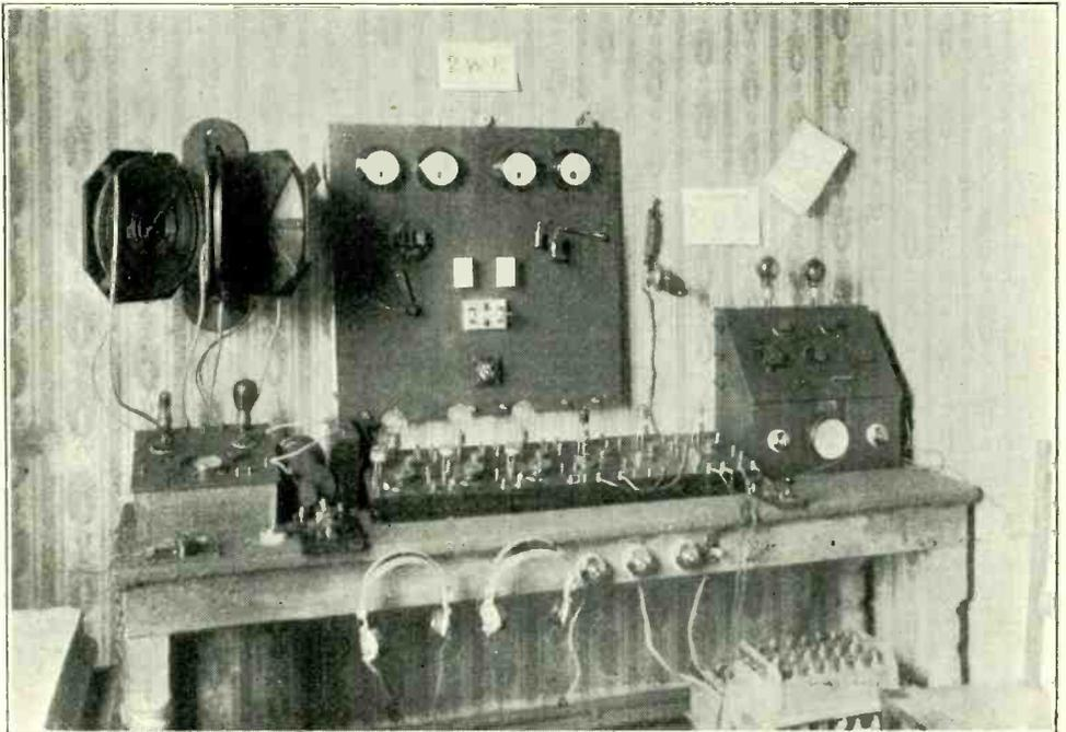
*The experimental transmitting and receiving equipment at 2WK, the station of Mr. G. R. Lewis.*
