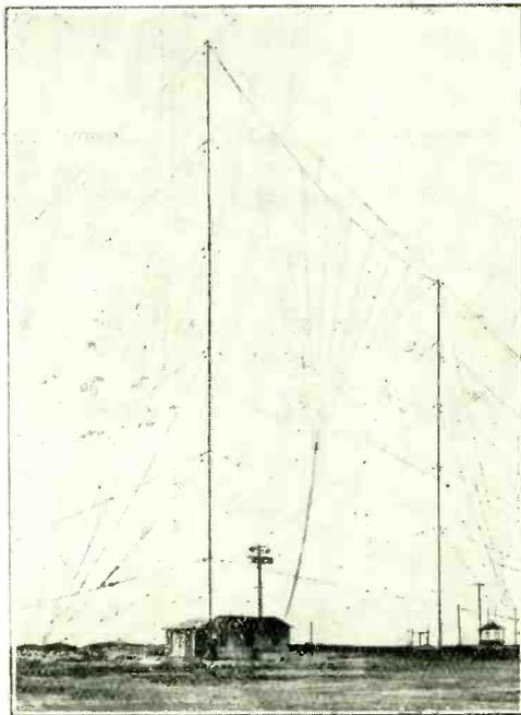
*The antenna at the Chicago Broadcasting station WJAZ. It will be observed that the fan-shaped aerial is suspended from an insulated wire attached to the two masts. The arrangement is particularly efficient for transmission on short wavelengths of 200 or 250 metres.*
