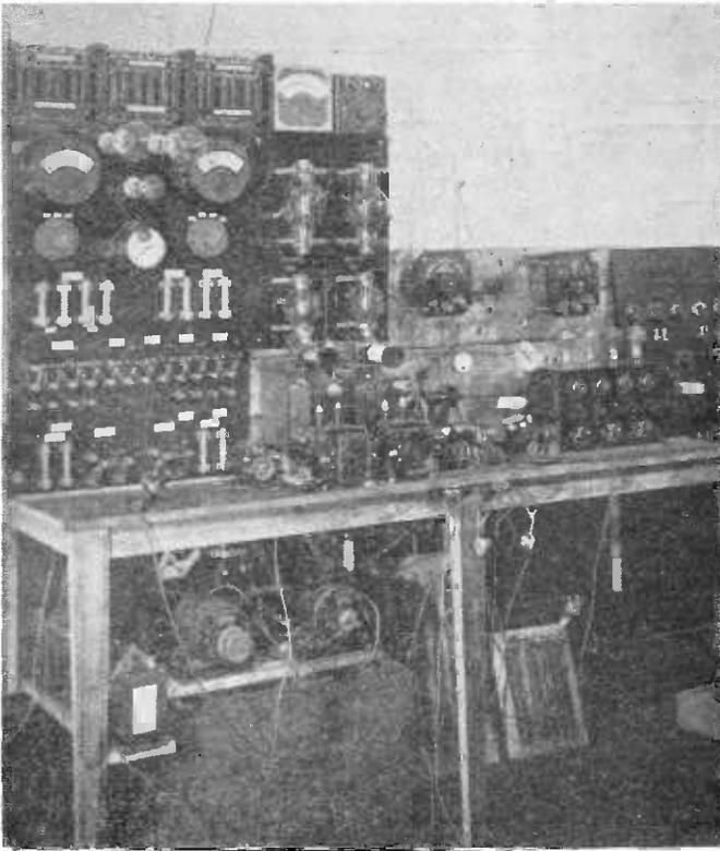
The experimental transmitting station (2 DY) of Mr. F. H. Haynes at Regent Square, London, W.C.1. The two small generators supply A.C. at 700 cycles for stepping up to H.T., and also for the filament heating of the rectifying, oscillating and modulating valves.
