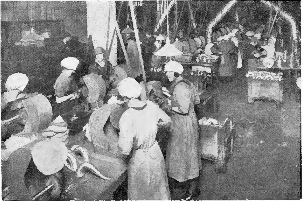
Loud-speaker horns passing through the polishing shop.
