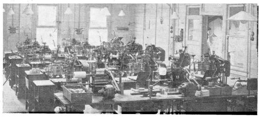
Some of the honeycomb duolateral coil winding machines at the Igranic Electric Co.'s works at Bedford.
