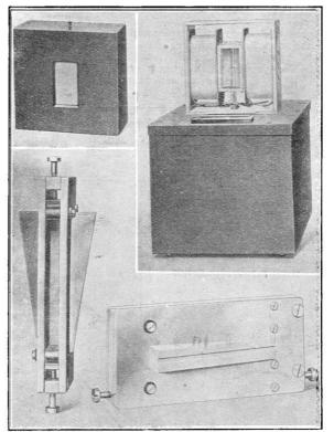
Fig. 3. Details of construction of the diaphragm. The upper right hand figure is a microphone operating on the same principle.
