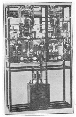
Courtesy: Marconi's Wireless Telegraph Co., Ltd. Suitable for either telegraphy or telephony, the Type U transmitter, seen above, Marconi operates on a power of 3 kilowatts.
