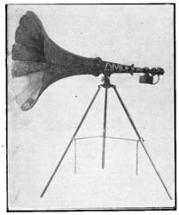
The loud speakers in use at the B.B.C. kiosk at Wembley are of the Amplion A.R. 49 type, of which the above is an example.
