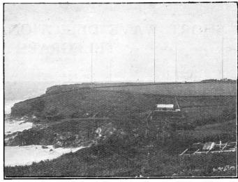
A distant view of Poldhu wireless station, between which and the yacht "Elettra," Senator Marconi carried out his short wave experiments. The four largest masts support the beam transmitting aerials.
