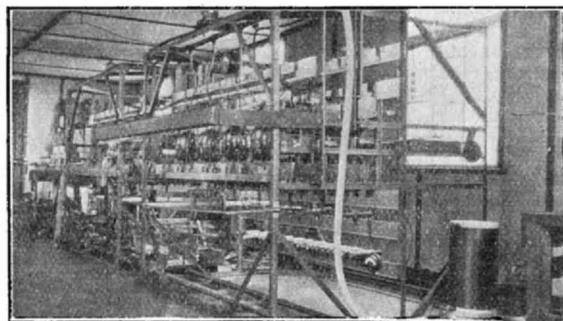
*Above : Short wave valve transmitting equipment at the Poldhu station.*
