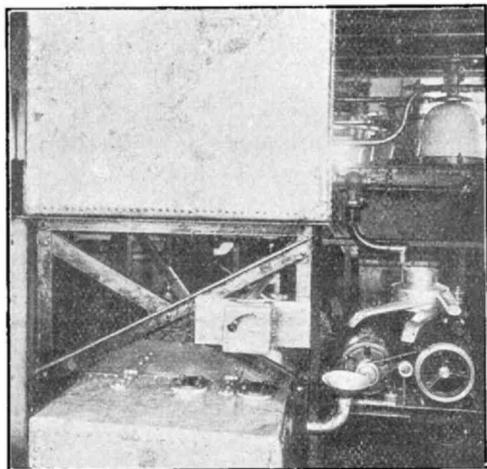
Fig. 5. Centrifugal separator and tanks.
