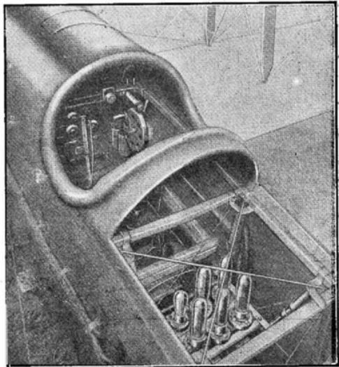
*The wireless equipment installed in an aeroplane.*
