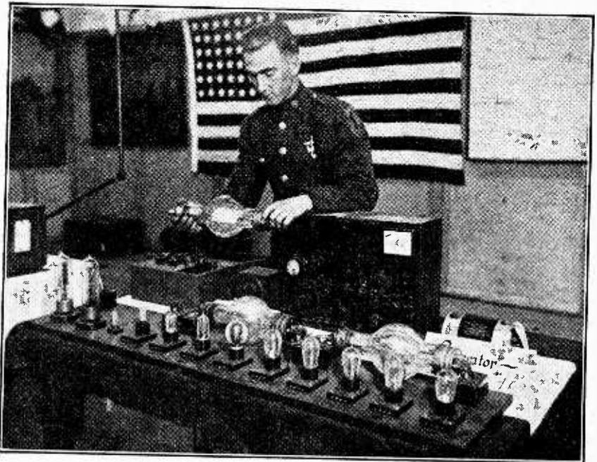
**A GAMUT OF VALVES.** A fascinating stand at the New York Radio Exhibition. This exhibit, arranged by the U.S. Army, showed every type of valve at present in use by the military signal service, from a tiny "peanut" to the largest 250 watt transmitting valve, taking 2,000 volts on the plate.
