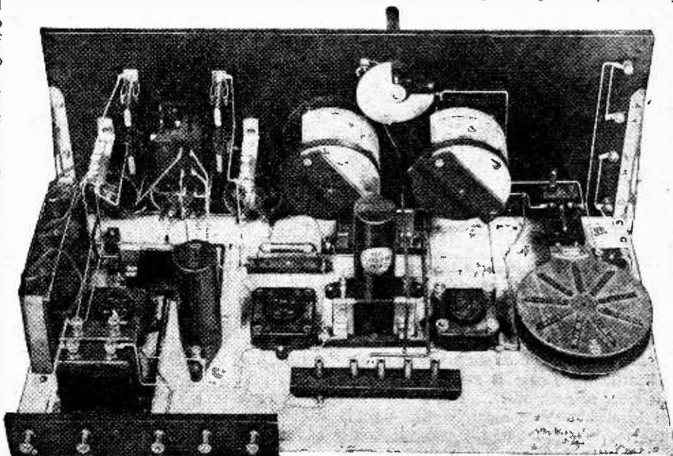
The receiver viewed from the back, with grid coil removed to show wiring of aerial and earth terminals and extra condenser sockets. The holder for the H.F. transformer is clearly shown.
