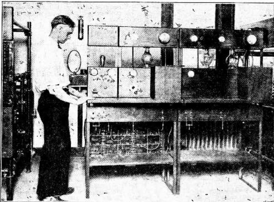
Crystal oscillator and amplifying equipment at KDKA.
