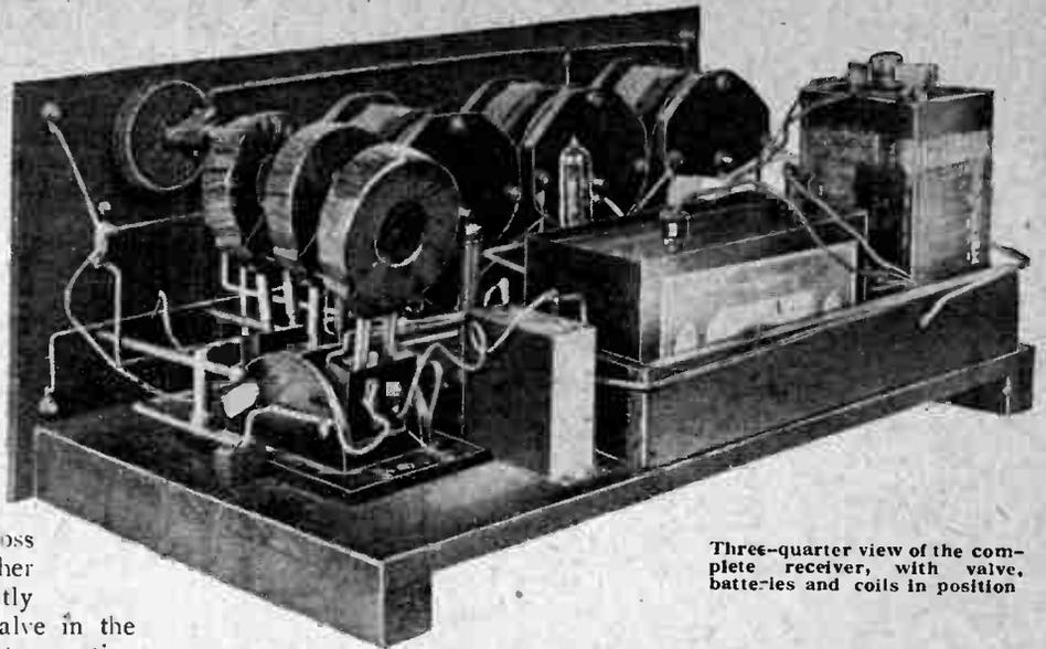
Three-quarter view of the complete receiver, with valve, batteries and coils in position
