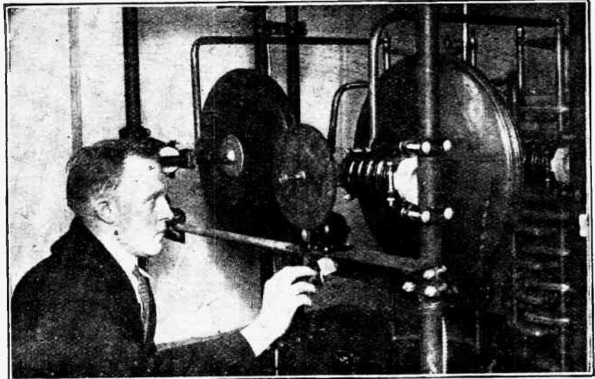
**THE LAST WORD IN VERNIER CONTROL.** This photograph, taken recently in the transmitting room of the 50 kW. broadcasting station, WJZ, at Bound Brook, N.J., shows the two variable air condensers used for fine tuning. Note the small electric motor which operates the condensers.
