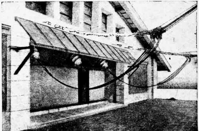
NO LEAKAGE HERE! The aerial lead-in at the high power station (PGG) at Kootwijk, Holland, which maintains communication on 9,000 metres with the Java station PKX. Owing to the terrific atmospherics in Java transmission has frequently to be made as slowly as ten words per minute.
