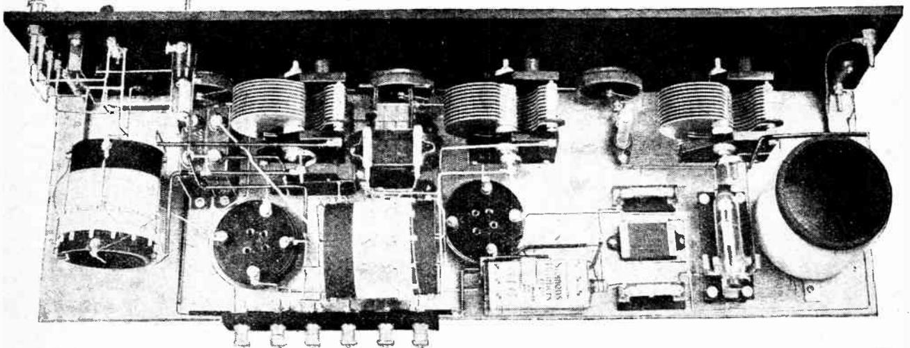
View from above. Note that the condenser C<sub>3</sub> is resting on the L.F. transformer, supported by its own wiring.
