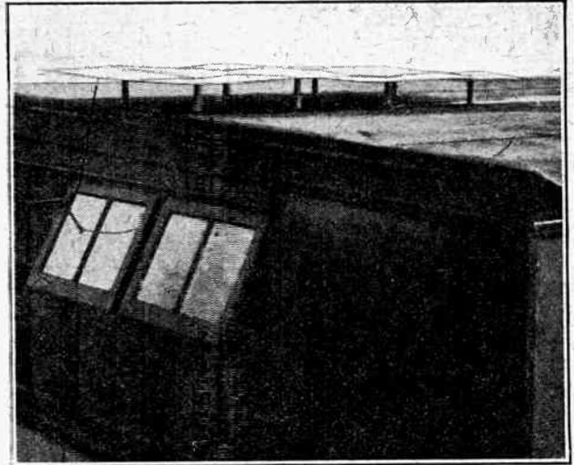
Aerial plate mounted on porcelain insulators on the roof of the receiving hut.
