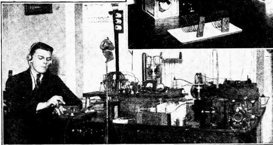
THE station of Mr. R. L. Royle, of Palmers Green, London, N., is well known to listeners on the short wave-bands. The receiving apparatus is here shown in detail, as well as a general view of the station equipment. It is to be observed that the lay-out is by no means elaborate, yet evidently capable of good performance. High-tension supply for the transmitter is derived from the alternating current mains, making use of an electrolytic rectifier.
