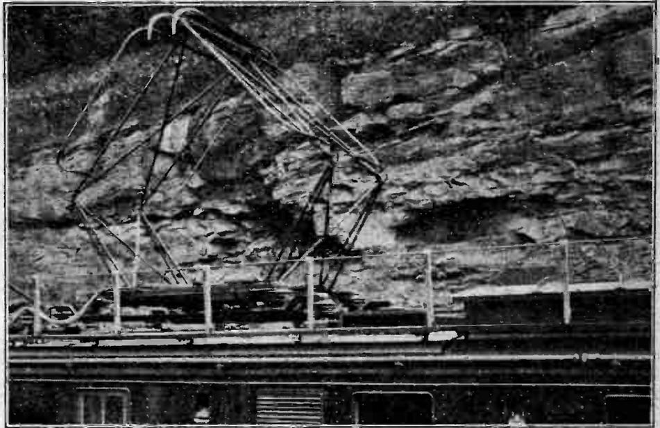
The cab roof of an electric locomotive on the Virginian Railway, showing the aerial mounted on porcelain insulators. The overhead power wires are used for carrier current signalling between the front and rear locomotives of long freight trains.
