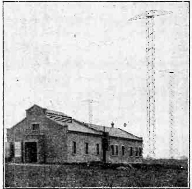
The newly-completed station building at Bridgwater, with three of the masts. Bridgwater is the beam receiving station, Bodmin constituting the transmitter.
