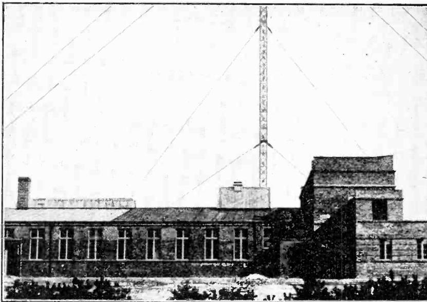
**WESTERN EUROPE'S BIGGEST STATION.**—Part of the station building and aerial at Zeesen, near Königswusterhausen. The new station, which uses a power of 40 kilowatts on a wavelength of 1,250 metres, will shortly supersede the original station at Königswusterhausen.
