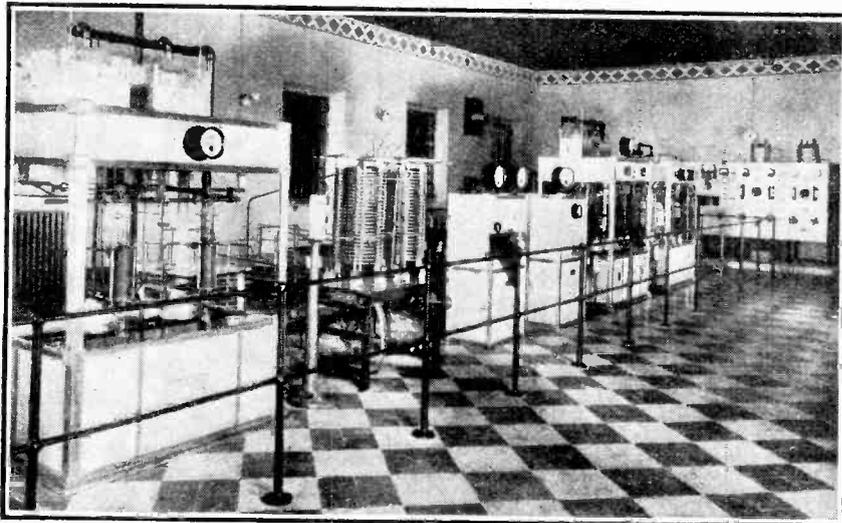
**BROADCASTING FROM ITALY.** Maximum efficiency is suggested by the spick and span appearance of the Milan transmitter, seen in the photograph. Built by the Marconi Company for the Unione Radiofonica Italiana, the transmitter yields an aerial power of 7 kilowatts. The main panels use water-cooled valves, the water being sprayed into tanks mounted on the top of the frames.
