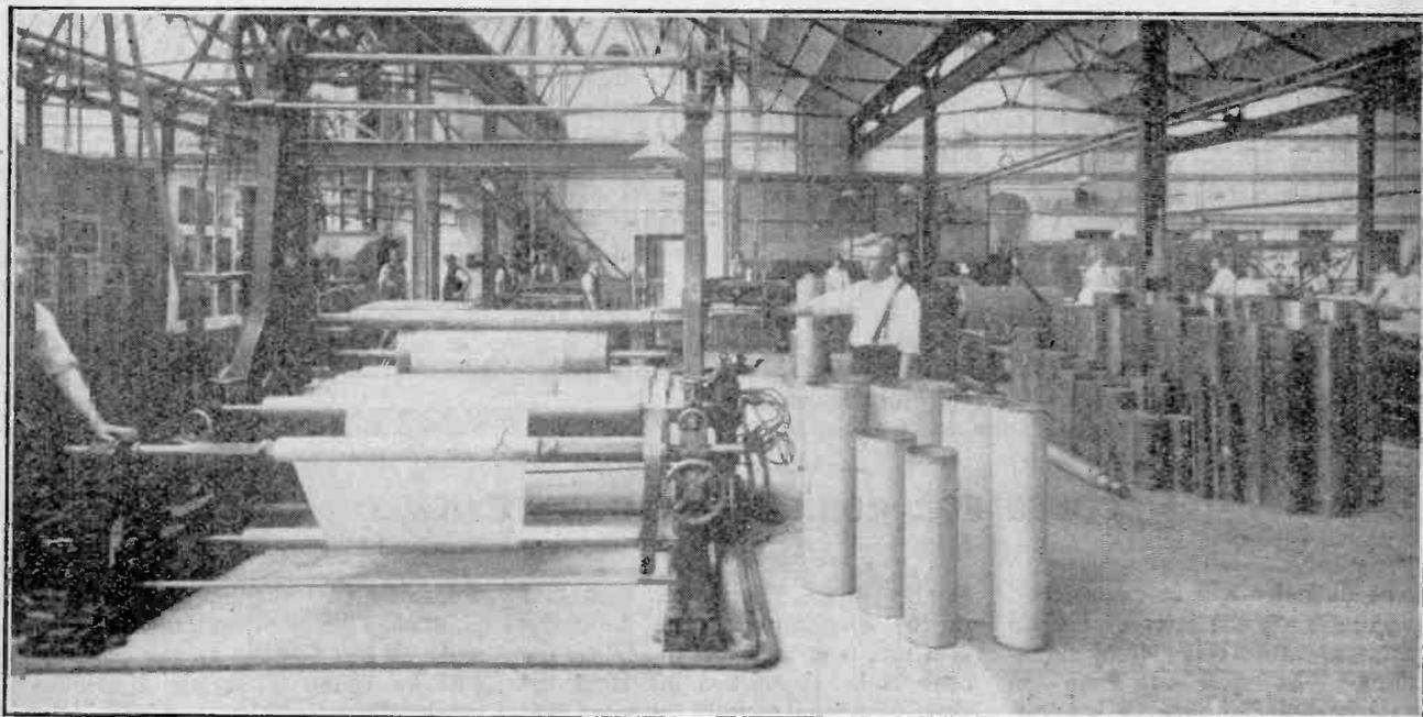
Fig. 4.—A tube-winding machine. The bakelised paper is slowly wound round mandrels against which electrically-heated rollers apply a heavy pressure.
