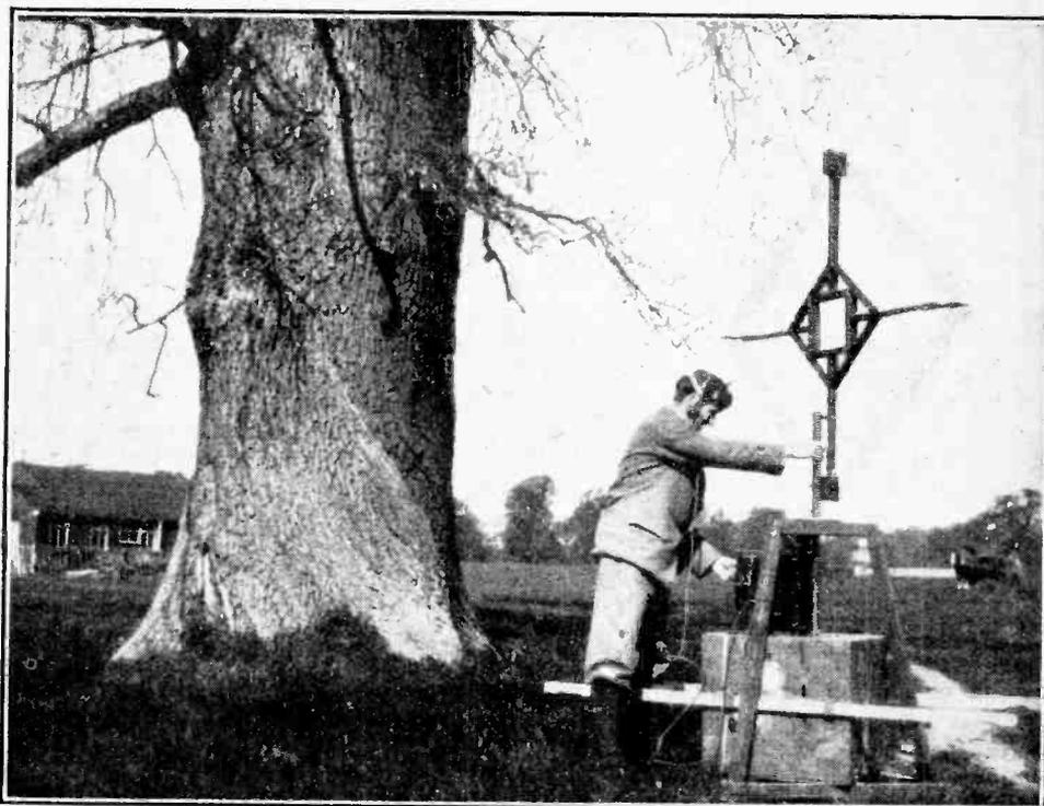
Fig. 6.—Direction-finding apparatus used in investigating the distortion of wave front by trees.
