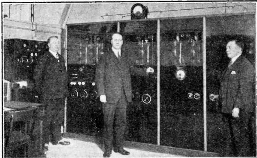
**A DANISH TRANSMITTER.** Engineers of the Copenhagen Broadcasting Station with the new Pedersen transmitter now undergoing nightly tests between midnight and 1 a.m. It will shortly replace the old transmitting plant, retaining the wavelength of 337 metres.
