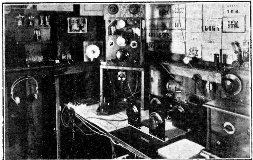
A NOTTINGHAM AMATEUR TRANSMITTER 2HD, owned and operated by Mr. Aubrey Harper at Cropwell Bishop, Nottingham, has been in touch with most European countries on wavelengths of 23 and 45 metres, and with an input of 4.5 watts. The transmitter shown is of the Hartley type. The receiver is a Reinartz.
