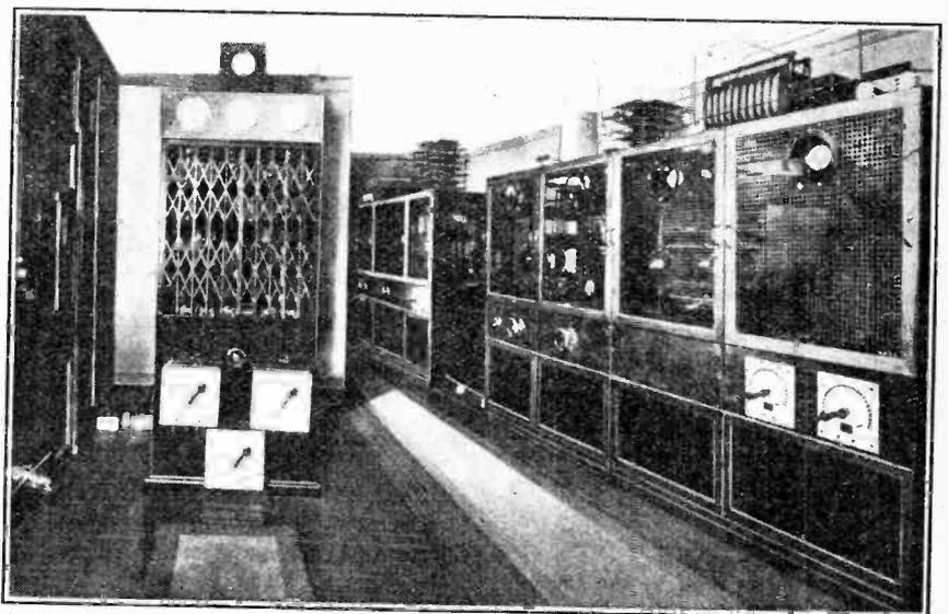
A POPULAR FRENCH STATION. The transmitting room at Radio Toulouse, showing the 5-kilowatt transmitter which is capable of working up to an aerial power of 9 kilowatts. Radio Toulouse celebrates its third birthday on April 15th.
