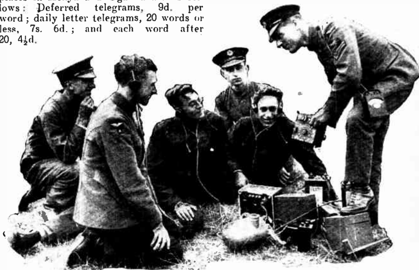
WAVEMETER MYSTERIES EXPLAINED. Members of the 600th City of London Squadron of the Auxillary Air Force (Territorials) receiving instruction in the use of the Townsend wavemeter.
