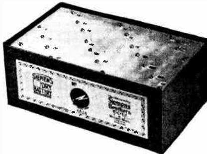
Siemens No. 1075 H.T. battery for portable sets.
