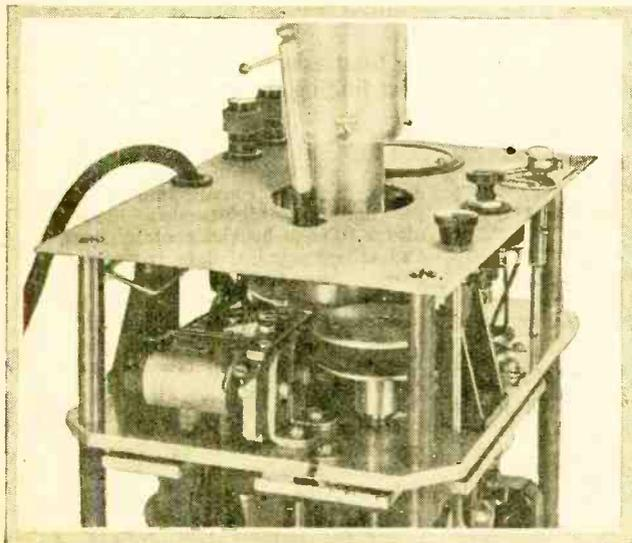
Close-up view showing the trigger release and driving pinion. One pole of the release magnet is hinged between centres.
