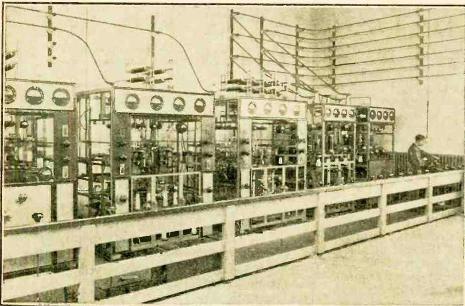
Oscillator and modulator panels of the 130kW. transmitter at Huizen, Holland, and (below) another corner of the station showing the rectifier valve panels.
