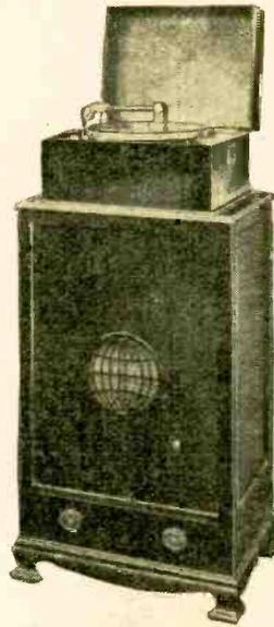
The Igranic electrically reproducing gramophone. Indirectly heated cathode valves are used in the early stages.
