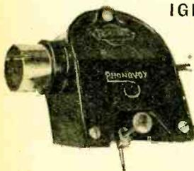
both cases and consists of a differential movement with the pick-up coil surrounding the armature, which moves between laminated pole pieces. In the tone arm model, however, the method of pivoting the armature is slightly different. The lower part of the armature is of square section and is bent at right angles to fit between two clamping plates lined
