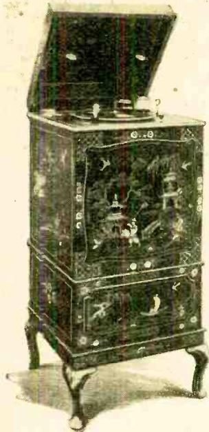
Celebritone electrically reproducing gramophone. An automatic trip cuts out the motor when the record is finished.
