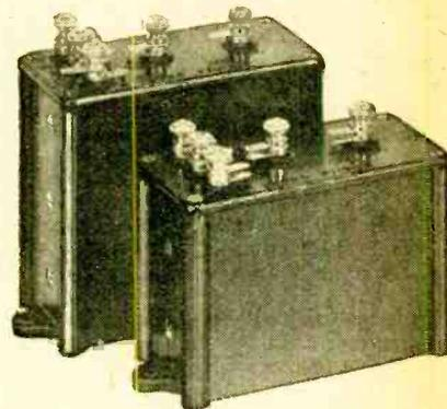
"Wearite" anode filter units. The larger size is for use in L.F. circuits.
