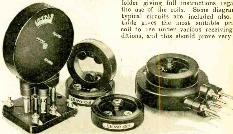
Lewcos "Super" six-pin aerial coils and H.F. transformers. The interchangeable primaries are shown in the foreground.
