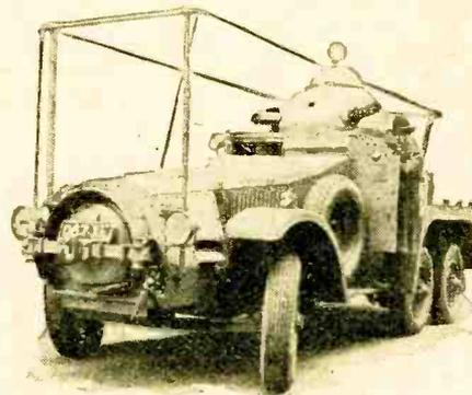
**ARMoured CAR WIRELESS.** A new type of car designed for patrol work on rough roads in India. The wireless transmitter and receiver can be operated on the move.
