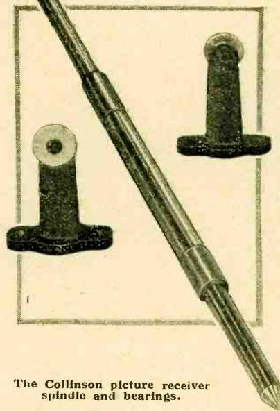
The Collinson picture receiver spindle and bearings.
