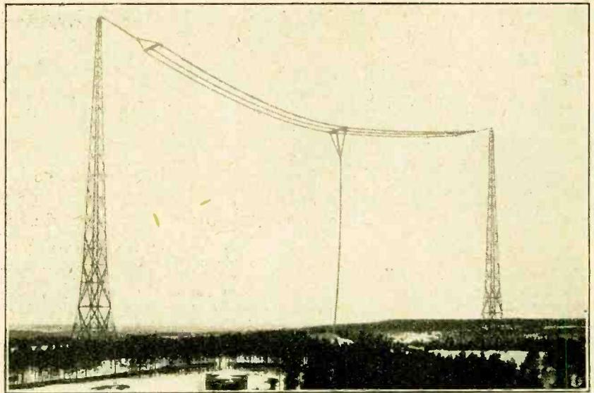
A CONTINENTAL GIANT. A general view of Finland's famous station at Lahti, which operates with 35 kilowatts on a wavelength of 1,504 metres.
