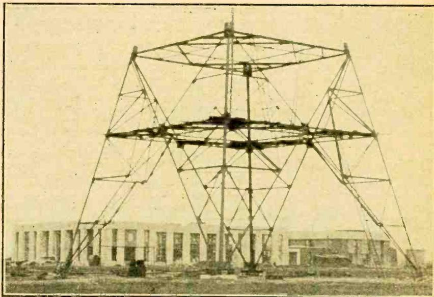
**LONDON REGIONAL.** The first photograph at Brookmans Park to show one of the masts under construction. It will be noticed that the mast is of the tritic self-supporting type—an innovation in B.B.C. practice.
