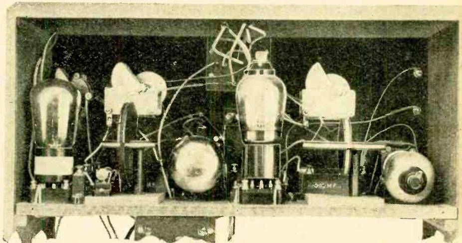
Short leads connect the switch with the frame sections. Wires are run by the shortest route between the components.
