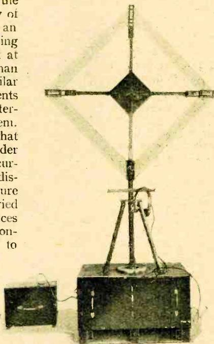
Fig. 1.—Single-frame coil direction-finder for wavelengths from 200 to 2,000 metres fully screened and ready for operation in making measurements of the strength of interference observed from high-voltage spark discharges.
