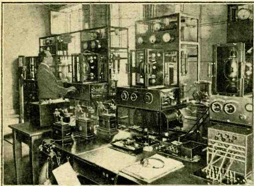
**THE STOCKHOLM TRANSMITTER**, which has an aerial power of 1.5 kilowatts. The station works on a wavelength of 438 metres. It supplies regular programmes to ten relay stations.
