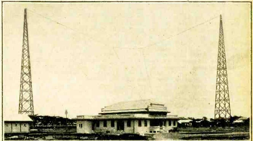
**SHORT WAVES FROM SIAM.** The Telefonken station at Bangkok. A double aerial is employed to permit of transmission on 14 and 17 metres without alteration to the tuning.
