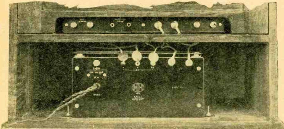
Back view of cabinet showing eliminator and H.T. and L.T. connections.
