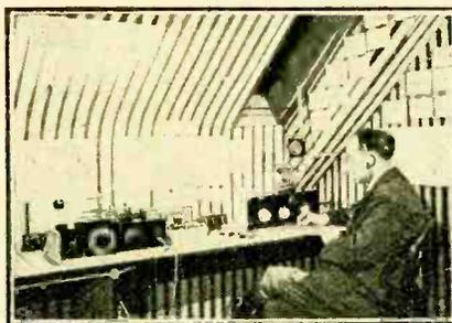
The French Amateur Station F8XZ at Saint Dizier, Haute Marne, has been in touch with most parts of the world with an input of 25 watts to a Colpitts circuit.
