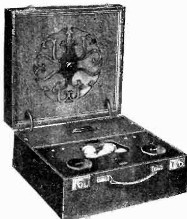
The Lissen portable to be found on Stands 184 to 186. A 5-valve receiver with one dial tuning.
