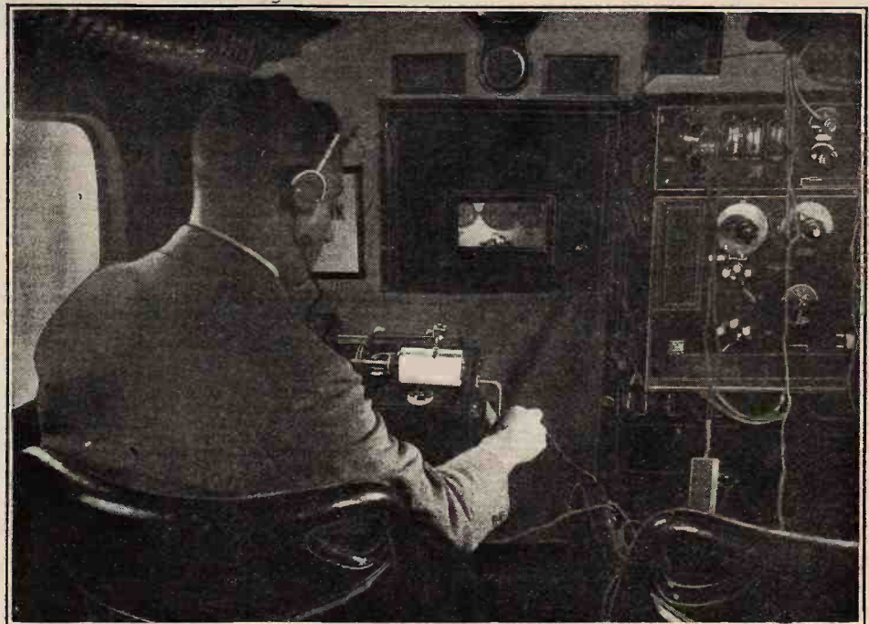
The Fultograph receiver in use in a Lufthansa aeroplane. To prevent spilling, a sponge soaked in potassium iodide solution was employed in the experiments. On the right is the Telefunken transmitter and receiver.
