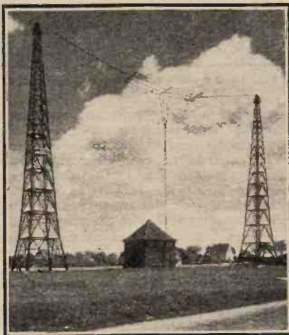
A STURDY RELAY STATION. Flensburg, which is heard at remarkable strength in this country although the power is only 0.5 kW. The station relays Hamburg on the common wavelength of 218 metres.
