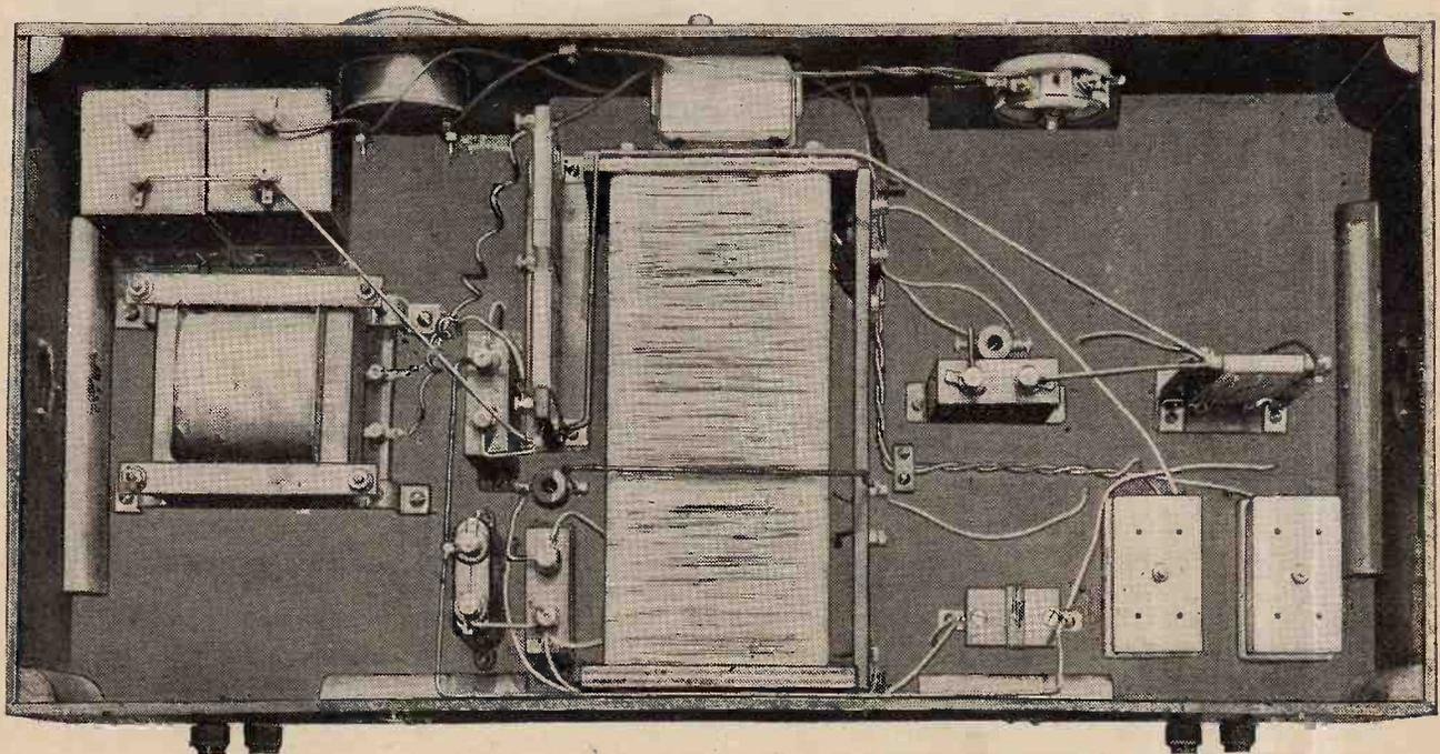
View of the underside of the sub-base showing the smoothing choke, voltage-regulating resistances and the 8 mfd. condensers on the left.
