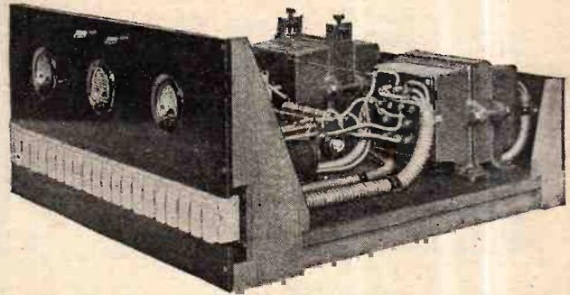
Mains equipment panel. Note the large number of fuses employed. Stray fields are prevented by carrying the leads in flexible metallic tubing.
