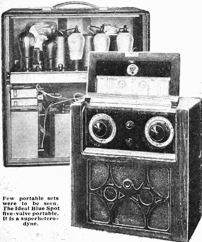
Few portable sets were to be seen. The Ideal Blue Spot five-valve portable. It is a superheterodyne.
