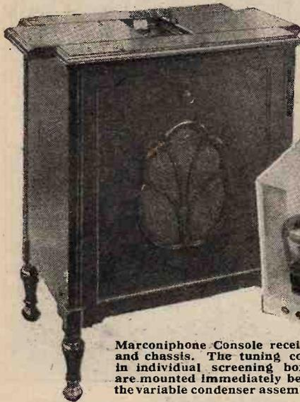
Marconiphone Console receiver and chassis. The tuning coils, in individual screening boxes, are mounted immediately below the variable condenser assembly.
