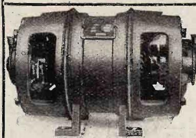
In order to show construction, end shields removed.
