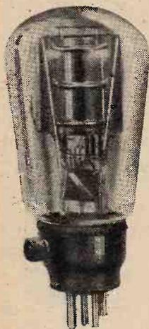
An indirectly-heated pentode—the Mazda AC/PEN.
