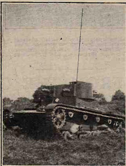
**A TANK AERIAL.** — This Vickers-Armstrong tank is equipped with a Marconi 8-metre transmitter, and the aerial consists of a flexible copper-plated steel rod, 12 feet high, which is almost invisible.
