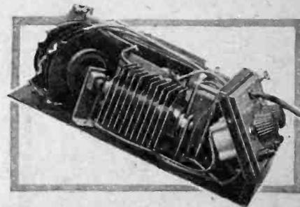
Internal arrangement of the eliminator components.
