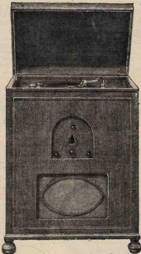
An All-electric Radio Gramophone for 100-120 volts & 200-250 volts, A.C., 40-60 Cycles.
