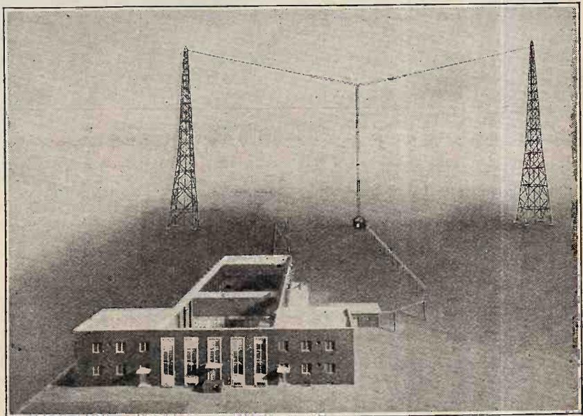
**ANOTHER GERMAN GIANT.** A model of the new high-power broadcasting station which opens to-day (Wednesday) at Heilsberg, Eastern Prussia, working on a wavelength of 276 metres and a power of 75 kilowatts. Like its companion station at Mühlacker, the new station can increase its output to 120 kilowatts.
