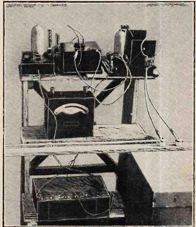
Fig. 5.—Experimental apparatus for investigating questions of modulation in connection with ultra-short waves.
