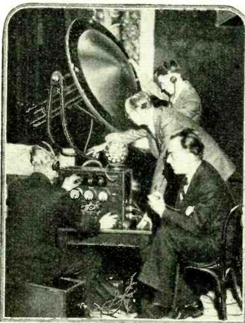
"FOCUSING" THE MICROPHONE.—Engineers of the American National Broadcasting Co. using a parabolic reflector microphone for an opera broadcast. The microphone is highly directional and can be turned towards any particular speaker, in the manner of a stage spot light.
