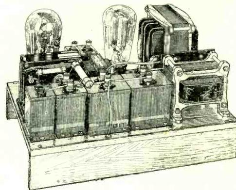
Power supply and output valve (250 volts) for the Monodial Super.
