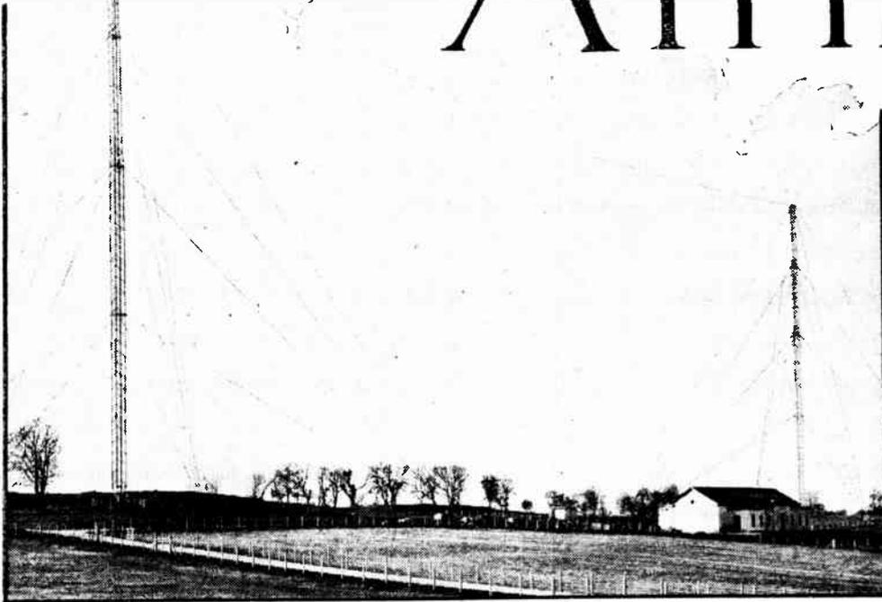
High power alone does not account for the excellence of the Athlone transmissions. The station is situated on an ideal site 300 feet above sea level, and the masts are 330 feet high.
