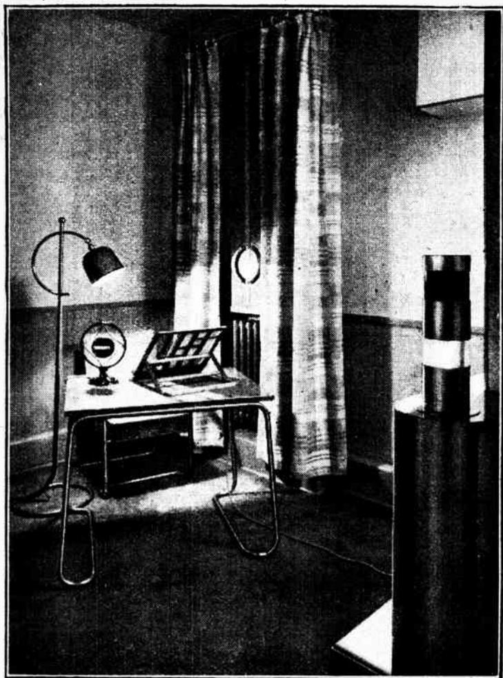
**WHEN LEEDS SPEAKS.** The talks studio at the new Yorkshire headquarters of the B.B.C. On the right is the "cue light" device for indicating to the speaker when the microphone is in circuit for broadcasting or, alternatively, connected to the dramatic control panel. The studio colour scheme is green and orange.
