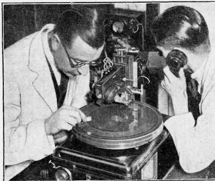
RECORDING THE KING'S MESSAGE. By special permission of His Majesty, an H.M.V. record was made of the broadcast message on Christmas Day. The engineers are shown superintending the recording on the wax blank, one checking the volume while his companion examines the sound track through a magnifying glass.
